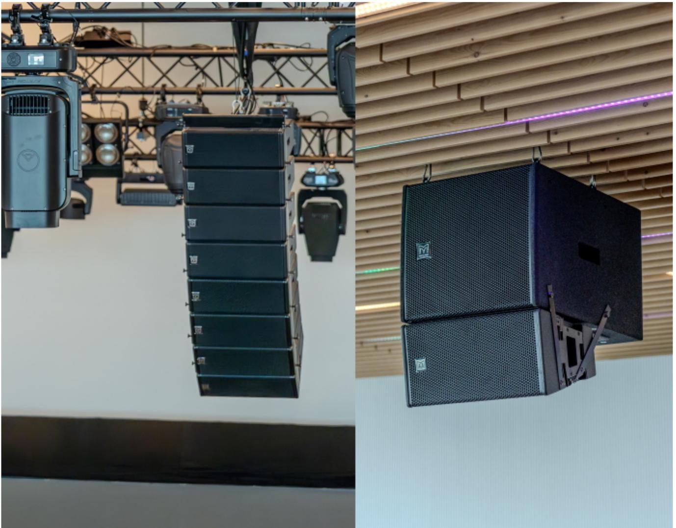
Complementing this is a delay of four TORUS T820 8" constant curvature speakers, providing defined 100° by 20° coverage pattern in the meeting areas at the mezzanine level, while four auxiliary CDD-LIVE 12 can be used as infills or outfills as required. Martin Audio's ADORN 5.25" ACS-55T ceiling speakers are set underneath the mezzanine to provide main system delays, or for independent use when this space is separated from the main hall - providing immense versatility.
