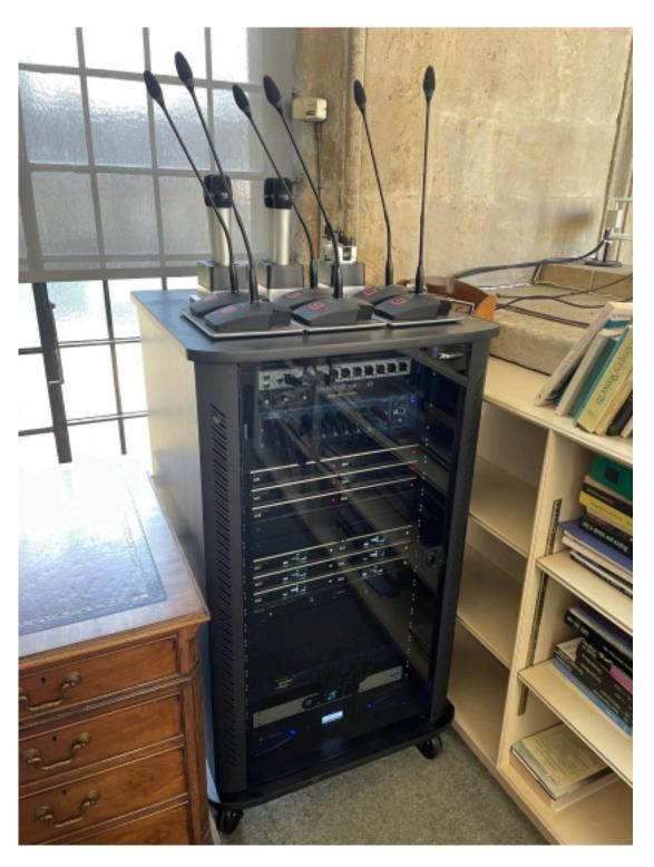
The SLDW system works with simple single button operation. Additionally, docking stations for charging have been mounted in a glass fronted rack unit, with speakers blending seamlessly into the room with a custom paint job. The easily accessible charging stations mean equipment is always ready for use and can last all day thanks to the 15 hour battery life.
