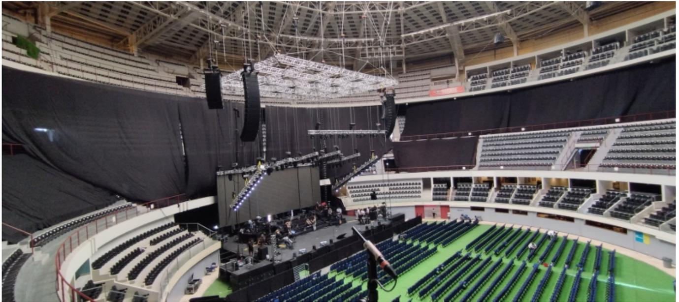
The full deployment at the GNP Acapulco Arena included 16 WPL per side for the main hang, run off iKON amps (in 2-box resolution), and eight MLA per side for outfill,. Subs comprised 24 SXH218 in an Inverted stack array. By designing it in a cardioid arc, it was able to cover 120° and provide a homogeneous and coherent coverage from the first rows to the farthest, right at the top of the venue. So complete was the coverage that only minimal front fill coverage was required.
