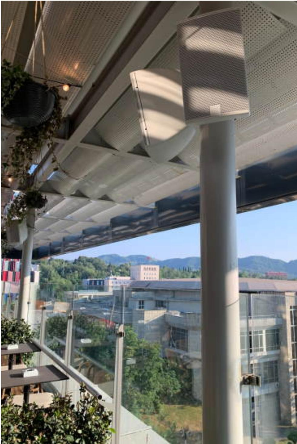
Inside, they have installed eight Blackline X8, and four SX112 subwoofers, flown from the ceiling. Outside they have opted for the weatherised CDD8-WR and CDD10-WR, with three SX112 sub enclosures ground-stacked.
