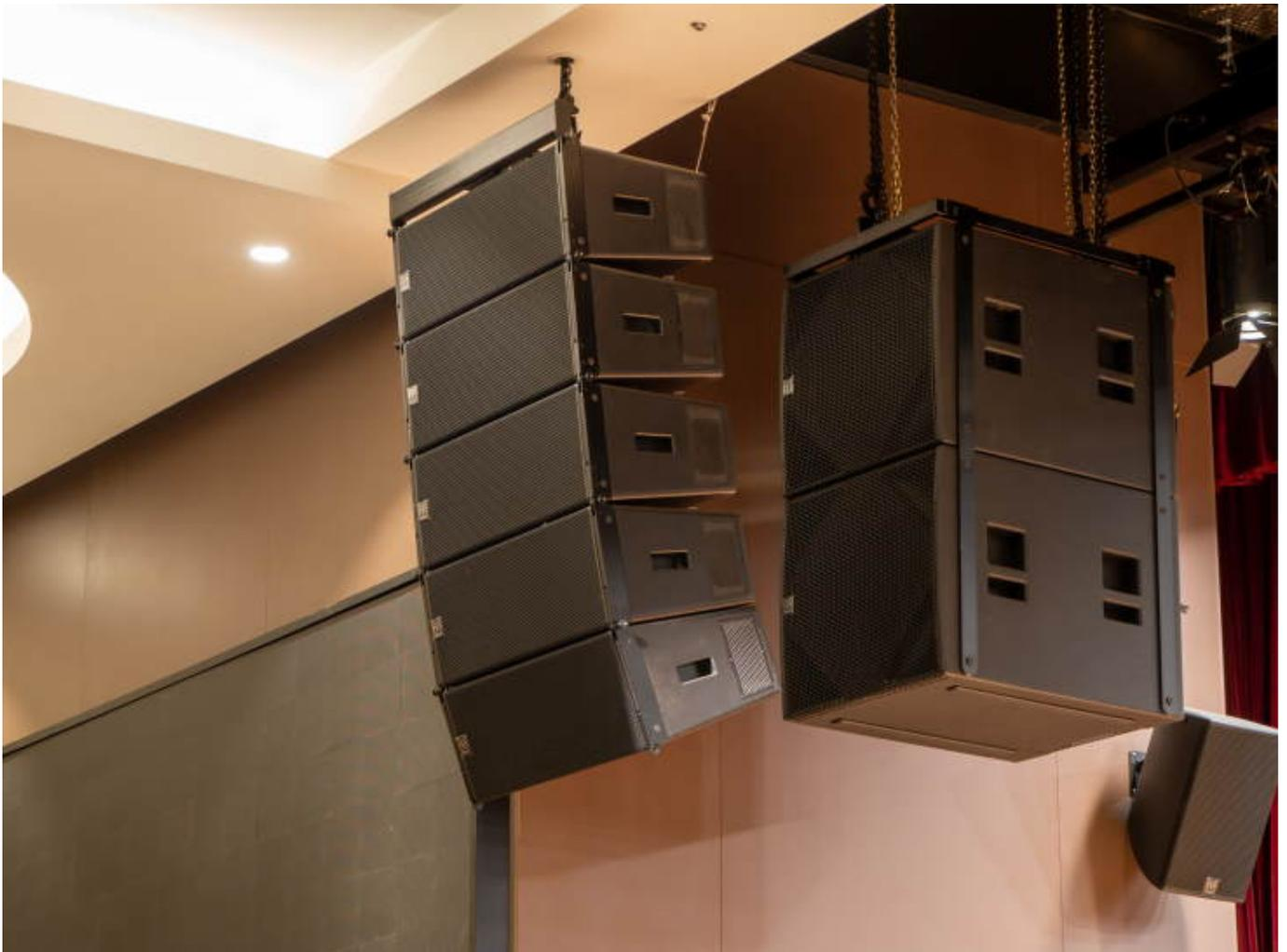
Set in hangs of five elements a side in the main Juniper Hall, accompanied by four SXC118 subs in cardioid, WPC is driven in 2-box resolution from an iKON iK81 and four iK42 amplifiers. A pair of LE200 wedges have been provided for stage monitoring.
