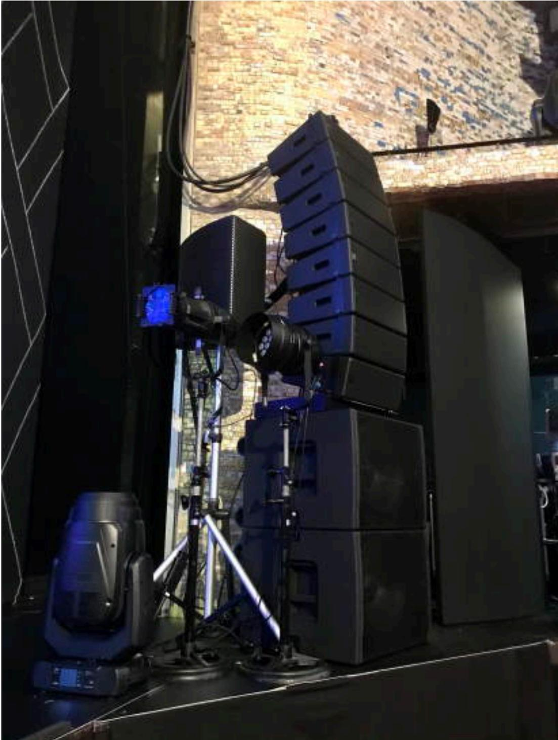
The theatre's installed proscenium L/C/R, along with wall speakers on the upper floor and second floor, those aimed at balcony seats, and a temporary Martin Audio ADORN A55 were set up in the back row of the second tier with a mic stand. In total, 31 outputs were controlled by a SARA II processor, the heartbeat of the Sound Adventures system.
