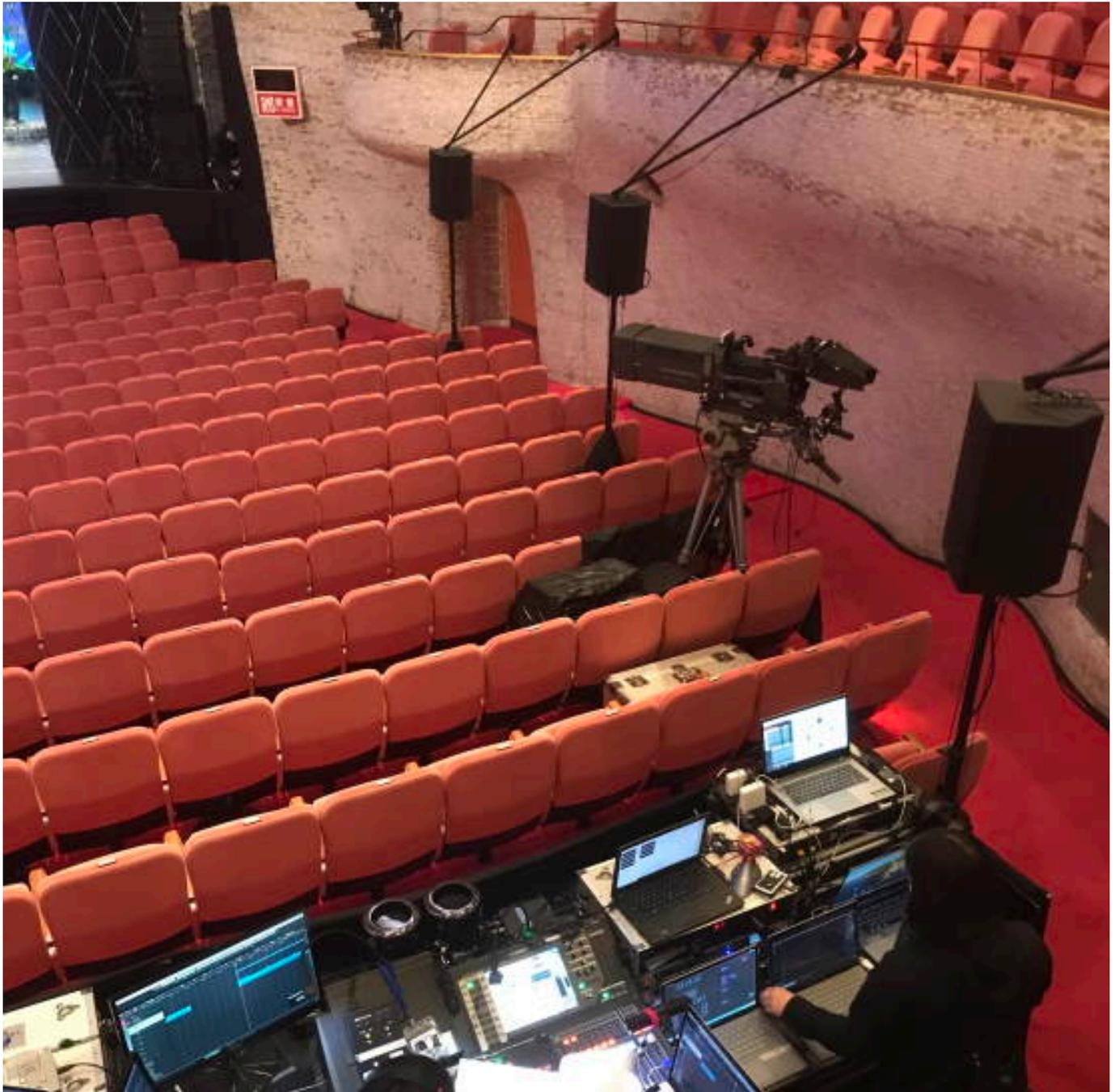
Martin Audio iK42 amplifiers were deployed to the WPM and XD12, and Lake LM44 processors were assigned to virtually all systems, to control both temporary equipment and permanently installed equipment - on the one interface - all connected by a Dante Digital Audio Network. Including the recording lines and backup Pro Tools, the number of Dante patch points exceeded 200.
