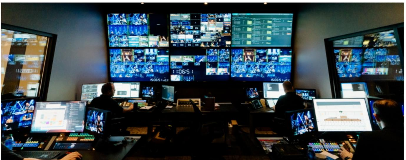
Eight FusioN IP converters at the edge convert IP signals to/from SDI and HDMI, enabling easy access to sources and displays. Twenty-one MuoNs inside a VirtU 32 frame, and other COTS switches, handle other signal conversion and processing, including the up/down/cross-conversion of HD and UHD. MicroN intelligent signal
